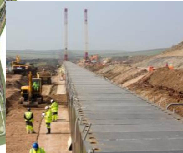
Holford Culvert - Complete
