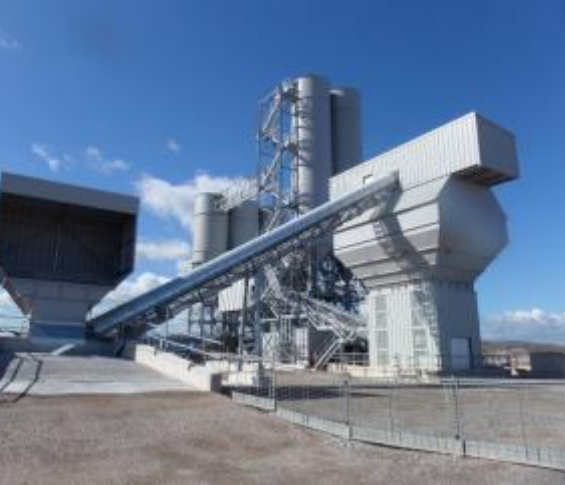
Batching Plant 1 - Complete
